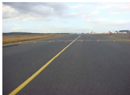
Examples of Apron Safety Lines and Passenger Path Lines
